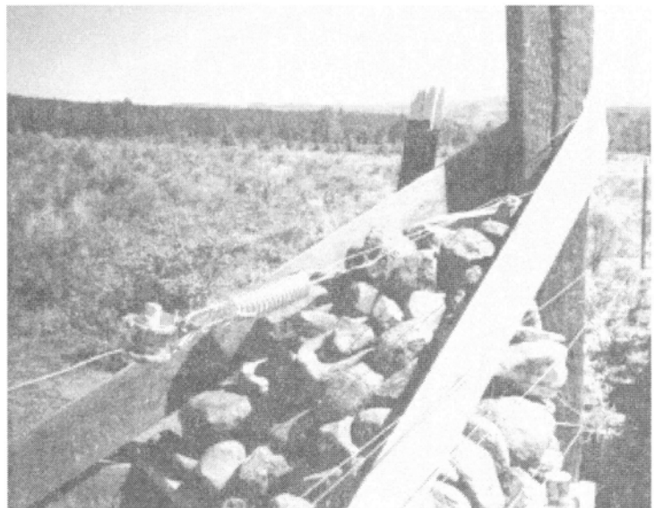
Figure 9 - 4: Water Gap Construction
